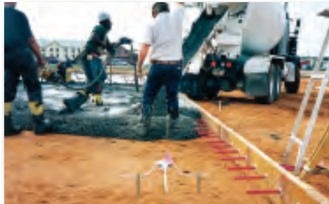
Step - 2 Make first placement of concrete
