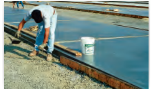
Step - 3 Strip form and insert dowel into SPEED DOWEL ®
