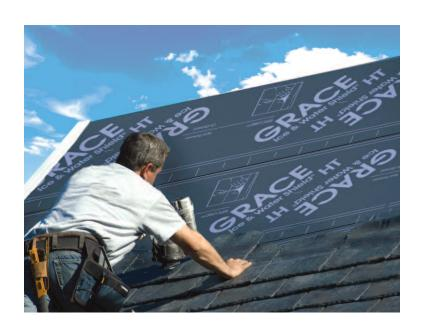
Reroofable—Unlike some granular surfaced membranes, Grace Ice & Water Shield HT will not adhere to the underside of the exposed roof covering. It can be applied over the old Grace underlayment (except over Grace Basik® except over Grace Basik®, Grace Tri-Flex® and Grace Tri-Flex® Xtreme™) in retrofit applications, making reroofing easier, less costly, more durable and environmentally friendly (as the structural deck remains intact avoiding the need to purchase additional wood decking).
