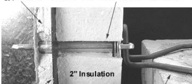
5/8" gyp-board 2-1/2" Pos-I-Tie® Self-Drilling Screw
