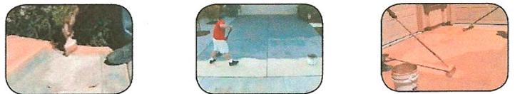
Use a bristle brush for edges and joints. Make sure that you re-broom the edges with the large applicator or a bristle brush or those areas could dry a slightly different color. If you get low on stain or run out, end on a joint. For large jobs or hot weather conditions, a second, wider applicator brush can help in re-brooming the stain.
