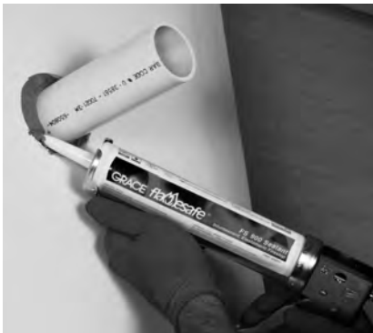
Metallic Pipe Through Concrete Floor or Wall – 3 Hour (UL C-AJ-1235)
