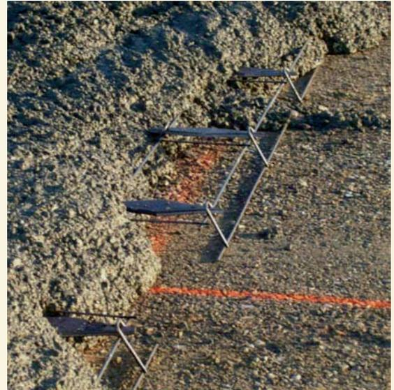
**Note:** Shipping wires need not be cut per the January 2005 American Concrete Pavement Association's *R&T Update*, "Dowel Basket Tie Wires: Leaving Them Intact Does Not Affect Pavement Performance".
