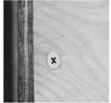
Plywood to steel or wood studs.
