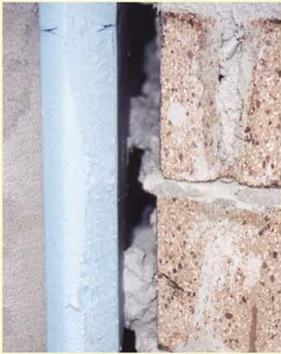
Figure 1 - Mortar Bridging
